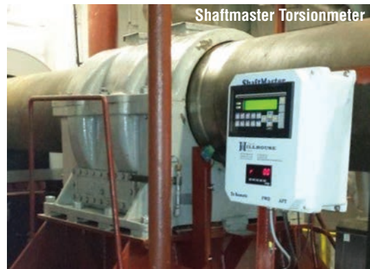
Standalone Rmp System that has (4-20 ma output) to the bridge and or control room to our touchscreen. Total, revolutions, direction and instantaneous Rpm for Maneuvering, Shaft Stop (optional) specific fuel consumption. Local and remote touchscreen bridge and control room viewed by 3.5” or 7 in” typical.
