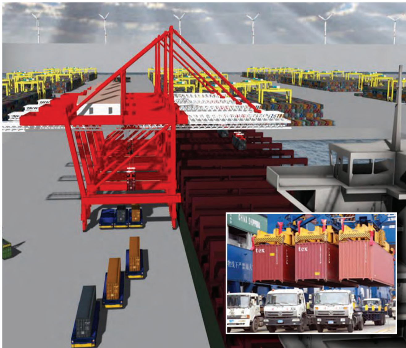
(LLNL photo: Inset photo courtesy ZPMC)
