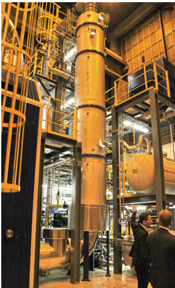
Left: View on the inline PureSOx scrubber arranged in the test facility. Right: The heart of the center: a MAN 9L28/32 engine which is coupled to a AvK-Generator with an output of 1,880 kW at 750 rpm.
