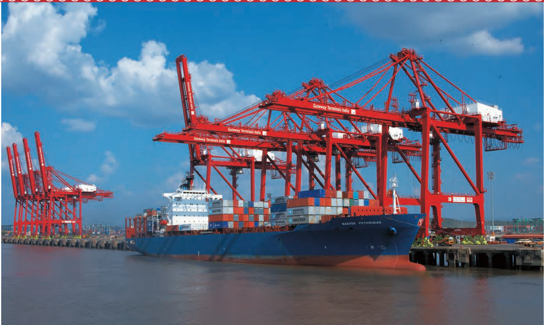
Gateway Terminal of JNPT - 1.
