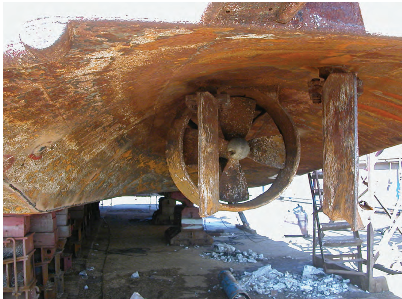
An example of a corroded prop and stern prior to a CP system installation.
