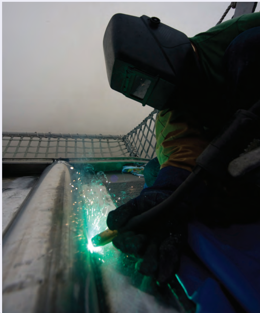
(Photo credit: Lewis Communications)
