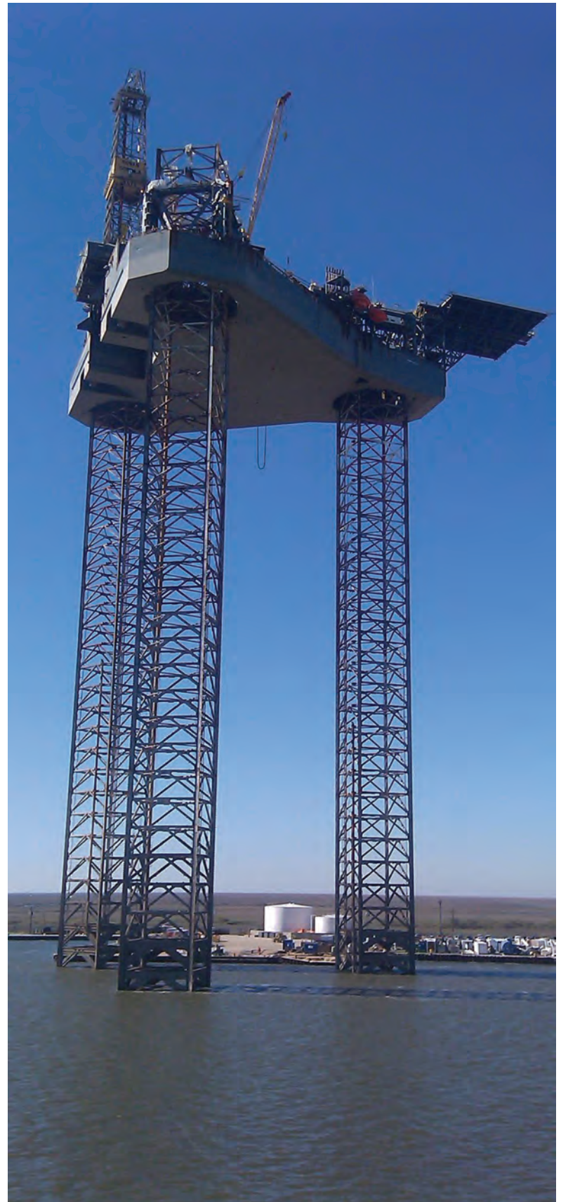
OFFSHORE STRUCTURES Rowan Gorilla IV adding legs at Rowan's Sabine Texas yard Photographed 2012 David Byrnes, Beaumont, Texas
