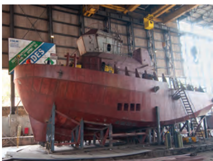
RAL Design under construction at the Estaleiros Rio Negro Ltda. (ERIN Shipyard) in Manaus, Brazil.
