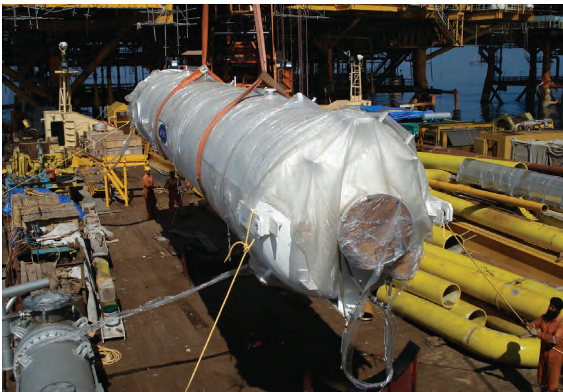
Installation of Separator of ICP Project.
