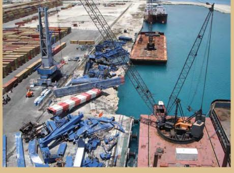
Mobro ABS barge mounted Ringhorse and American 11320 (450t) crawler lifts collapsed container crane from water in Freeport, Grand Bahama.
