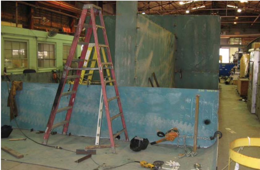
Hurley Horn Insert being constructed.
