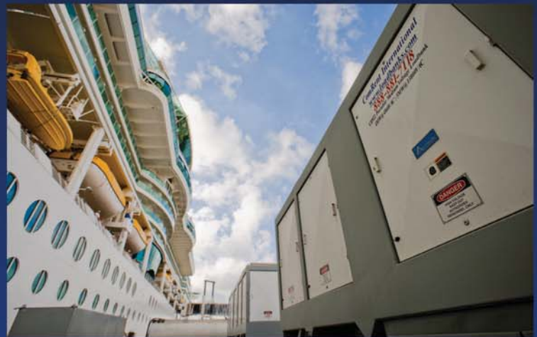
CR922 Medium Voltage Load Bank
