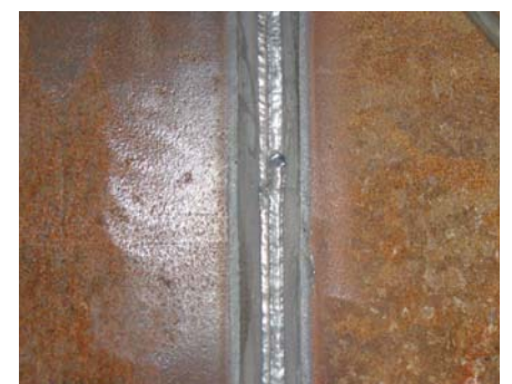
Shown here is the welding of a root seam and cover pass created with Miller's PipePro 450 RFC and the Regulated Metal Deposit (RMD) technology.
