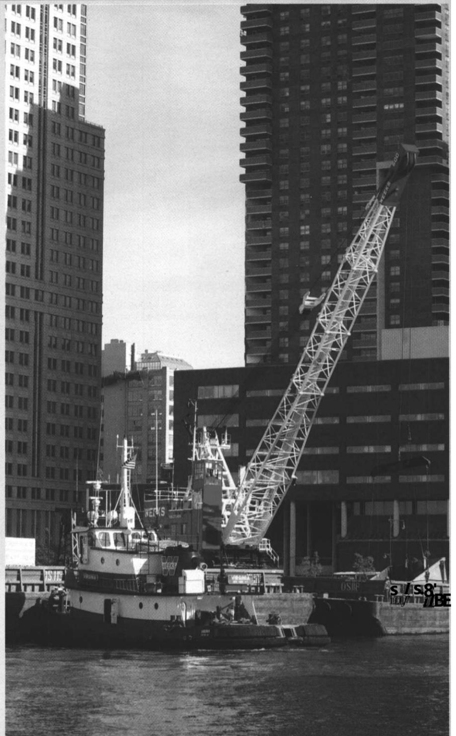
A crane, a tug, and barges at the emergency loading site created at Pier 25, N.R. Here, this and a second Weeks crane transfer WTC scrap and debris from trucks to the barges, for disposal elsewhere around the port of New York. (Photo: Don Sutherland.)
