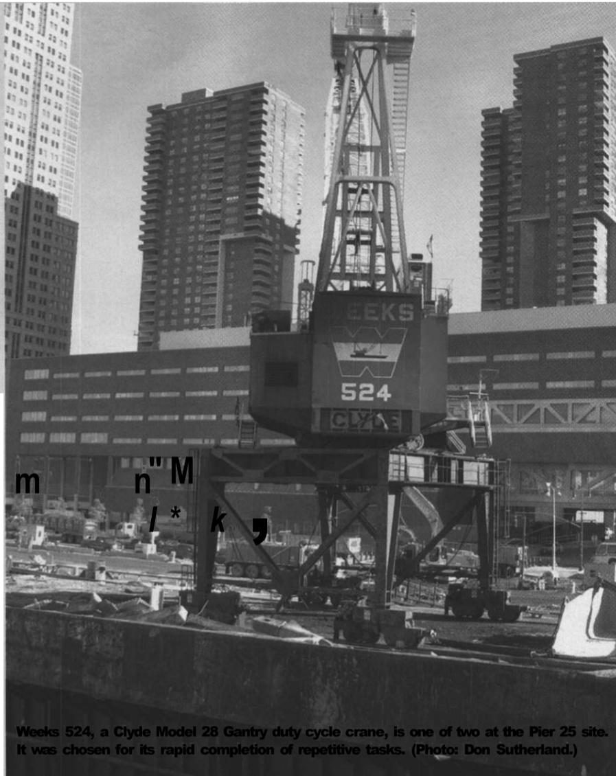
Weeks 524, a Clyde Model 28 Gantry duty cycle crane, is one of two at the Pier 25 site. It was chosen for its rapid completion of repetitive tasks. (Photo: Don Sutherland.)
