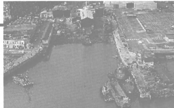
Astilleros Zamakona is just one small shipyard, which reaped huge savings in materials, production and design hours by integrating a computerized 3-D modeling system.
