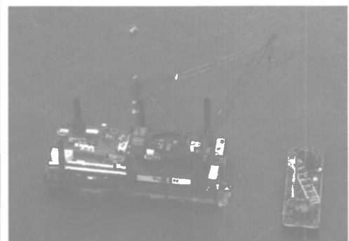
An aerial view of Karlissa-B preparing to lift suction piles and lifting truss from the deck of a material barge.
