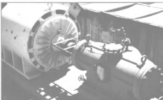
2 Fuel Oil Transfer Pumps Size 8x6 Mfg: DeLaval
