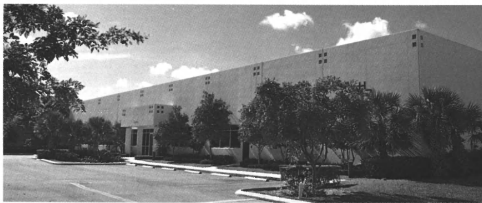
Existing Facility In Deerfield Beach, Florida - Circa 1993
