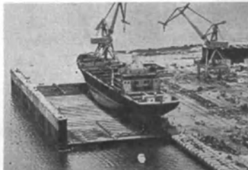
2. In this view the ship has been moved onto the launch platform from shore to platform by means of a special transfer distance is about 300 feet and required four hours was moved at a rate of 22 inches a minute. The platform
