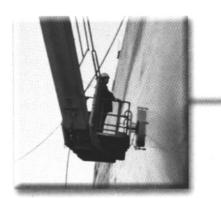
Rotating SPIN JETs<sup>®</sup> make short work of cleaning or preparing large surfaces.
