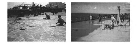
Surface preparation by hydrojetting, spotblasting where necessary, followed by high pressure washing with fresh water. After drying, application of 2 coats of Jotamastic 87 then 1 coat of Penguard Topcoat.
