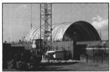
from the sun in summer, and minimizing wind chills and keeping out rain and snow, during the winter. The covers are customfitted to any drydock, and are made in two, three, four or more movable sections, with each section retracting to 35 percent of its extended length. Two people can open and close the sections in minutes, or if required, the retractable cover may be engineered to move with electricity or air located on the drvdock.
