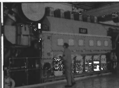
The Caterpillar CM43 engine was designed for drillship applications.
