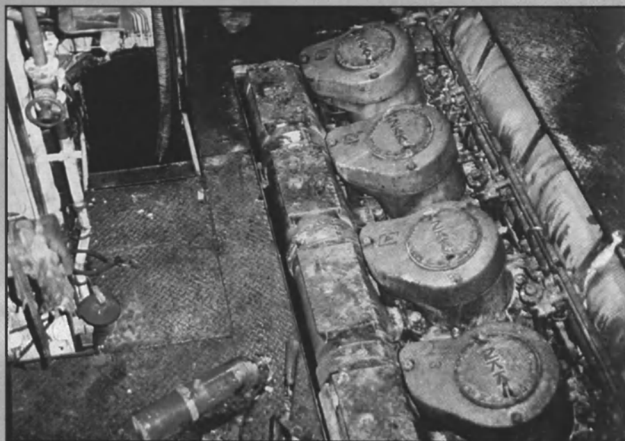
Pictured above is the aftermath of an engine room fire.
