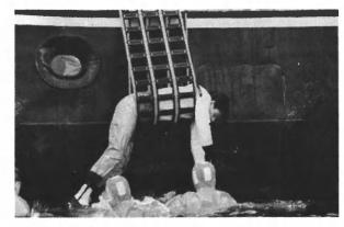
JASON'S CRADLE forms a par-buckle, giving the rescuer a 2:1 mechanical advantage. In most situations, once the casualty is placed in the non-colapsial legop, the recoverage coss takes 4-8 seconds
