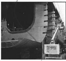
The recent conversion of FPSO Glas Dowr was also carried out by Harland & Wolff with the assistance of the company's Repair division. The project included major engineering work and the complete fabrication and installation of a helideck.
