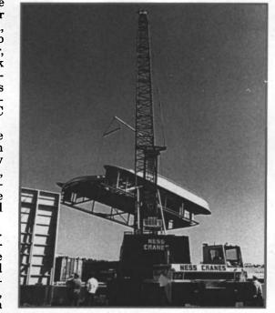
The thin plate and complicated structure of the *Navatek II* superstructure illustrates the type of plates and shapes prepared by Northwest Plasma Cutting. Northwest Plasma Cutting's M.G. cutting machine is located in a high bay building with overhead cranes and truck-wide doors to facilitate handling of raw and finished plates and shapes.
