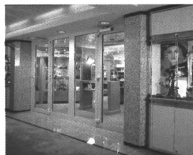
• Fire Rated Glass; Sprinklers
