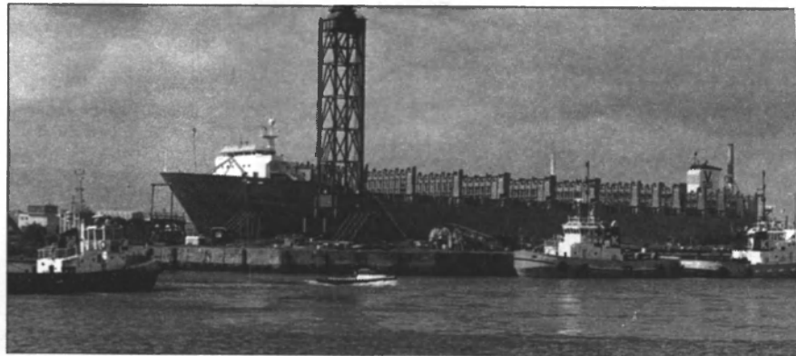
A hatchless containership built at Verolme Heusden and fitting out at Wilton Fijenoord.
