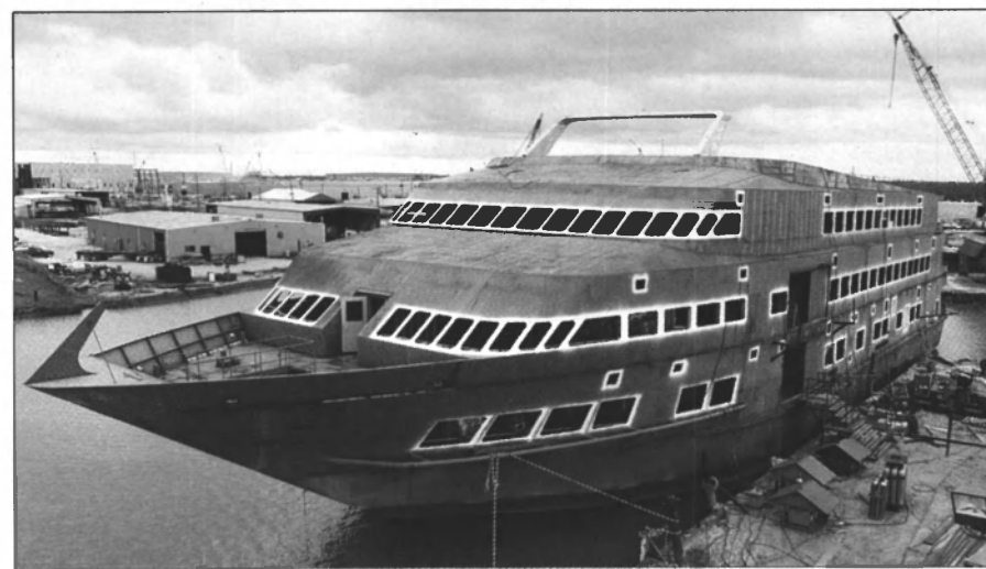
Harrah's Casino boat under construction at Service Marine
