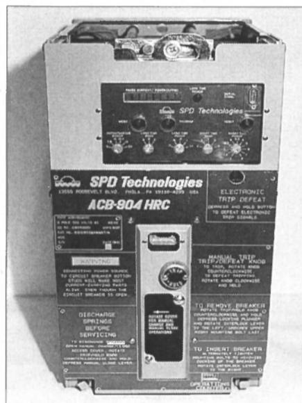
The ACB-904 circuit breaker, the first 900 amp circuit breaker with electronic overcurrent protection.
