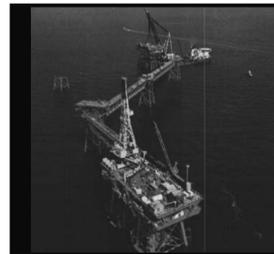
McDermott's DB50, rear center, sets Production Platform No. 1 deck for Freeport-McMoRan Resource Partners (Limited Partnership) Main Pass Block 299 Sulfur Project in the Gulf of Mexico, completing the western one-third of the 15-platform offshore sulfur mining complex.
