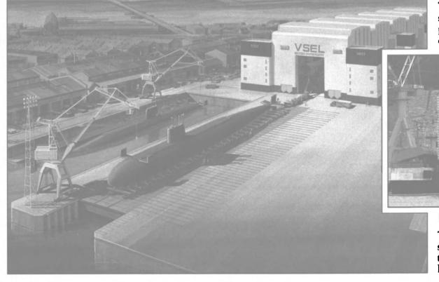
The greatest lifting capacity shiplift in the world – 24,000 tons for nuclear submarines at Barrow-in-Furness, England.
