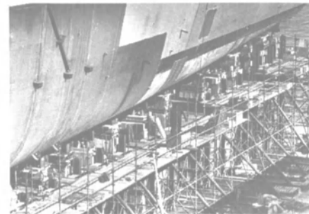
The OTC Power Team hydraulic jacking system is visible in this view of USS Roberts.
