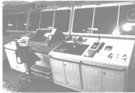
The M/T Petrobulk Mars can be operated safely by one person on the bridge day and night under normal operating conditions.
