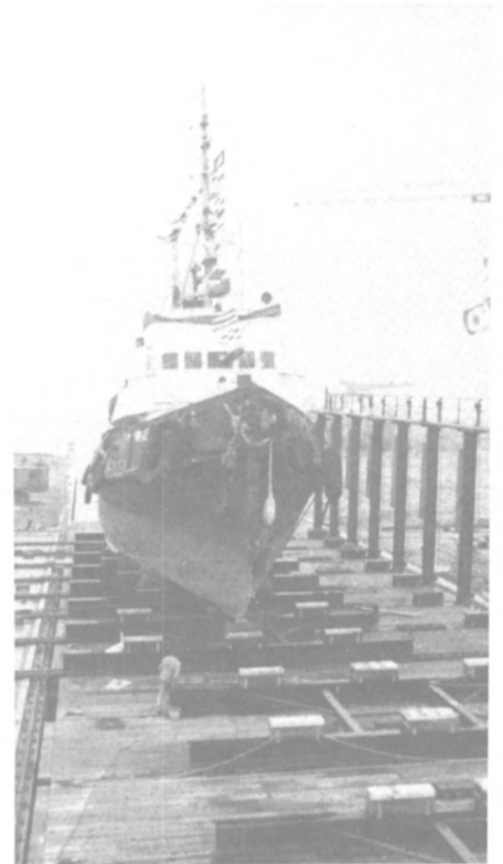
Crandall-designed 1200 ton railway dry dock.
