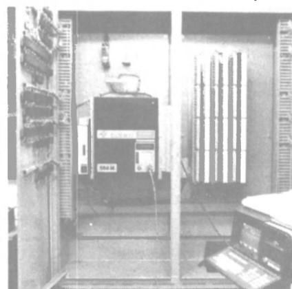
Alarm and control panel (ACP) aboard the Bobo showing Modicon 584M mounted inside left compartment. Right compartment contains I/O unit for the ACP.
