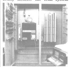
Alarm and control panel (ACP) aboard the Bobo showing Modicon 584M mounted inside left compartment. Right compartment contains I/O unit for the ACP
