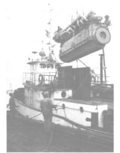
The Stork-Werkspoor 9FHD-240 diesel engine being lowered into the Brenda H.
