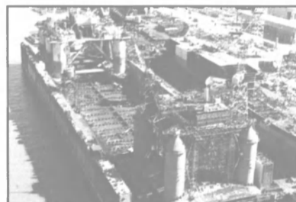
2 rigs in 900-foot length, 220-foot width inside wing walls of dock.
