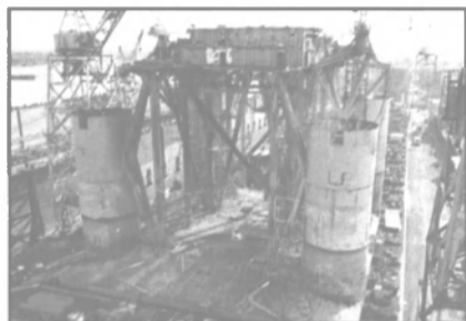
Column removal, deckhouse rebuilding.
