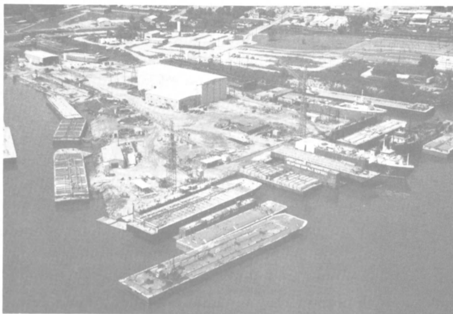
Newpark's yard on the Houston Ship Channel
