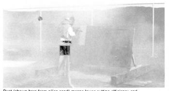
Dust (shown here from silica sand) means lower cutting efficiency and visibility and increased health hazards and clean-up costs.
