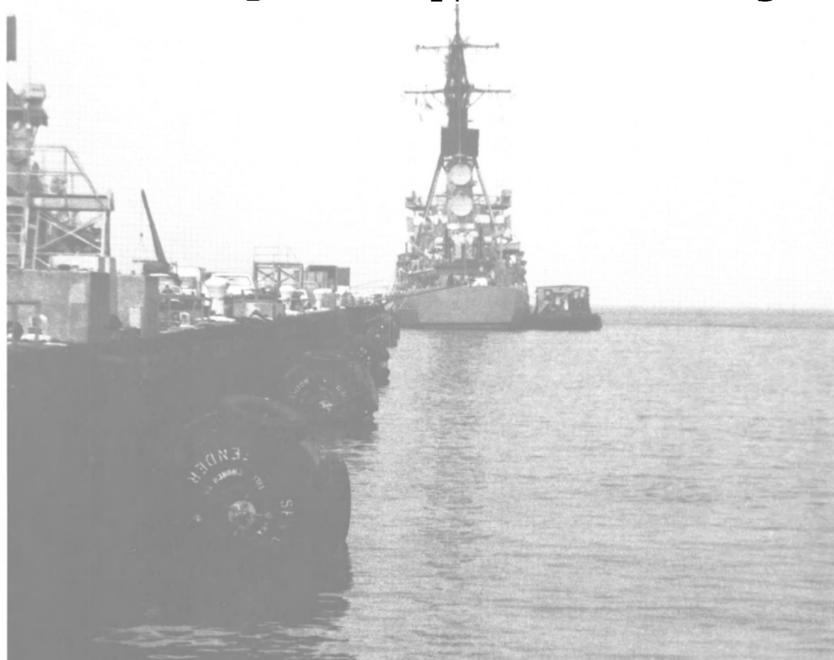
Prior to installing SEA CUSHION foam-filled fenders, the U.S. Navy was spending millions of dollars each year to replace broken fender piles at its piers. Many times this amount was also being spent to repair ship hull damage caused while berthing.
