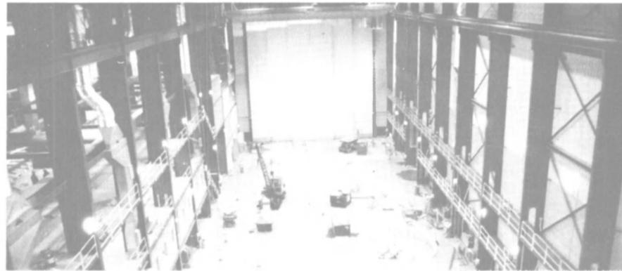
Gangways from the mezzanine on the left and from walkways on the right provide quick access to ships under construction and eliminate the need for traditional scaffolding. At the front and rear of each bay, 70-foot high doors, consisting of 6 sliding panels, open to a width of 65 feet.
