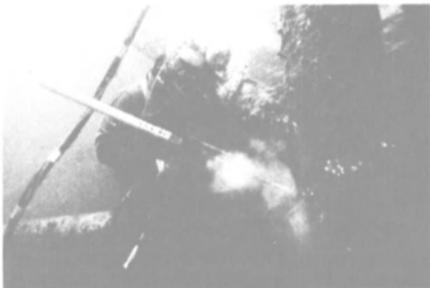
Barnacles and marine growth can be easily cleaned with 20,000 psi on land or by using a zero thrust gun underwater.
