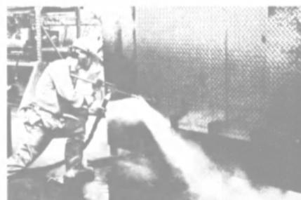
Rusted surfaces are cleaned to "near white" metal.
