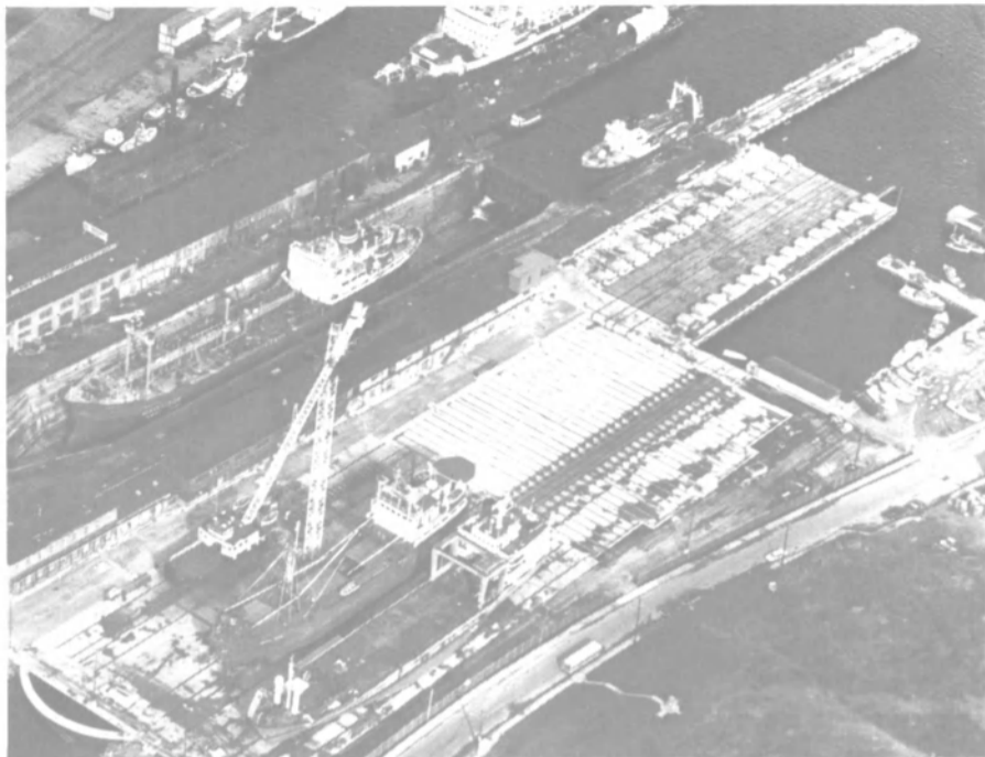
Recent aerial view of Newfoundland Dockyard shows (from top right) the Syncrolift ship elevator, the side-transfer table, and the three new repair berths. The graving dock shown, which was placed in service in 1926, will continue in use.
