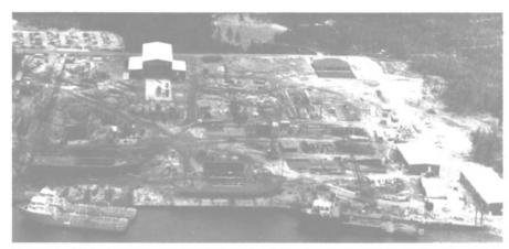
Moss Point Marine's modular construction system enables a vessel to be constructed in different sections simultaneously on their 21-acre site on the East Pascagoula River.
