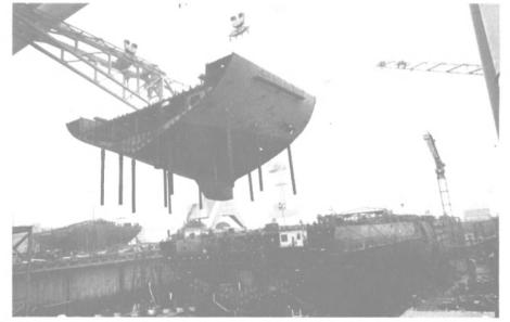
Newport News Shipbuilding made history when it successfully lifted an 890-metricton assembly onto the aircraft carrier Theodore Roosevelt (CVN 70) under construction at the shipyard with a 900-metric-ton-capacity Krupp crane.
