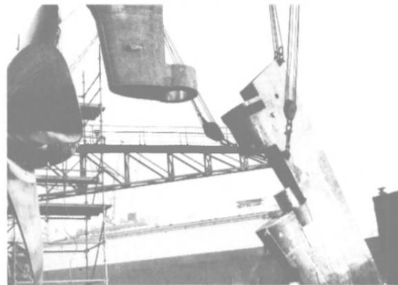
The repaired rudder is ready for hoisting at Wilton-Fijenoord shipyard, part of the Wilton-Rotterdam Dockyard Group, Netherlands.
