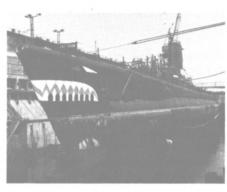
"FISH" OUT OF WATER - The USS Torsk submarine, built at the Portsmouth Naval Shipyard in New Hampshire in 1944 and the last submarine to fire a torpedo and sink a ship during World War II, gets a routine drydocking for testing, cleaning, and painting at Bethlehem Steel Corporation's Baltimore repair yard. The Torsk now is a tourist attraction in Baltimore's Inner Harbor and drew 96,000 visitors
