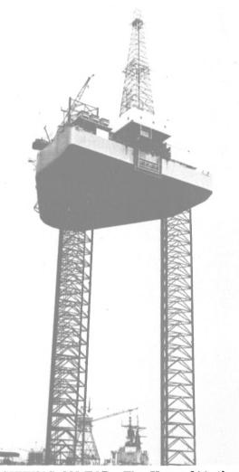
SITTING ON TOP—The Keyes 301, the second L-780 self-elevating offshore drilling unit to be built for Keyes Offshore Companies, Houston, Texas, by Ingalls Shipbuilding, Pascagoula, Miss., is jacked to the top of its 390-foot legs during successful testing operations prior to recent delivery. The unit is now drilling for ARCO Oil and Gas Company off the Louisiana coast. Ingalls, the third largest rig builder in the country, has 14 additional units under contract, including two more for Keyes.
