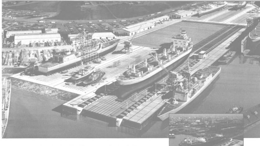
Todd Pacific Shipyards Corp., Los Angeles division, has just become the newest member of the Syncrolift family . . . now 148 installations in 58 countries. When completed, the Todd Syncrolift will be the largest shiplift in the world . . . 655 feet long, 106 feet wide, with a lifting capacity for vessels up to 48,000 DWT. An adjacent transfer system will enable the yard to service five maximum size ships ashore at one time.
