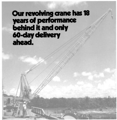
Those are two major advantages to consider about the Levco 360° 5-ton revolving crane. In addition, it's easy to service by your own mechanics and most parts are galvanized or inorganic zinc coated for complete protection against corrosion.
