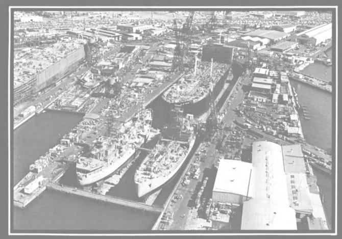
NASSCO's  $1000' \times 175'$  graving dock being fully utilized to build the first of three 37,500 DWT Carlsbad Class Product Tankers for Union Oil and to reactivate/re-engine two Alatna Class T-AOG gasoline tankers for the U.S. Navy (MSC).
