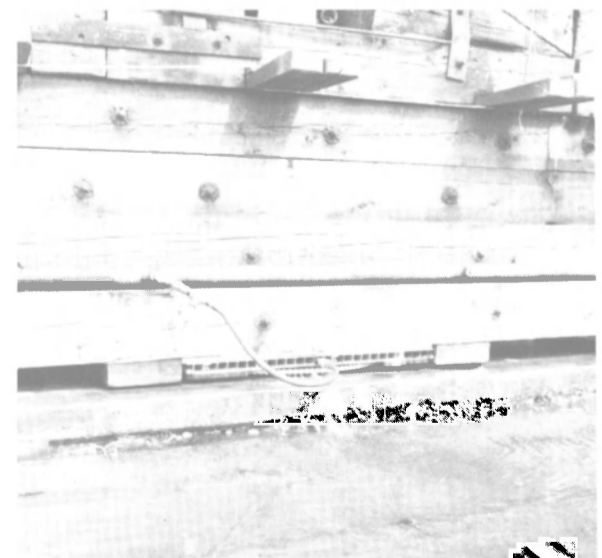
Typical water bearing installation under the barge shoring.
