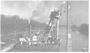
1. Gatelifter, 500 ton lifting capacity, electrically controlled, c/w upright steam boiler, 160 lbs. steam pressure capacity. Engine: W.H. Allen & Sons 290 BHP 400 RPM, 10" stroke, 12½"×22" cylinder. Generator: 200 K.W. 240 volts, 833 amps, 400 RPM. Mounted on Moulded Hull Barge, 62' wide, 90' long, 26' deep, 15' draft, overall height water line to ton of boom 120'. top of boom 120'. Location: St. Catharines, Ontario
