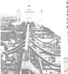
MINIMUM OUT-OF-SERVICE TIME. Modern equipment achieves blasting and coating rates for 2-coat epoxy on normal surfaces in the range of 2,000 square meters (20,000 sq. ft.) per day using experienced American and Hispanic personnel.
