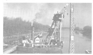
1. Gatelifter, 500 ton lifting capacity, electrically controlled, c/w upright steam boiler, 160 lbs. steam pressure capacity. Engine: W.H. Allen & Sons 290 BHP 400 RPM. 10" stroke, 12½"×22" cylinder. Generator: 200 K.W. 240 volts, 833 amps, 400 RPM. Mounted on Moulded Hull Barge, 62' wide, 90' long, 26' deep, 15' draft, overall height water line to
