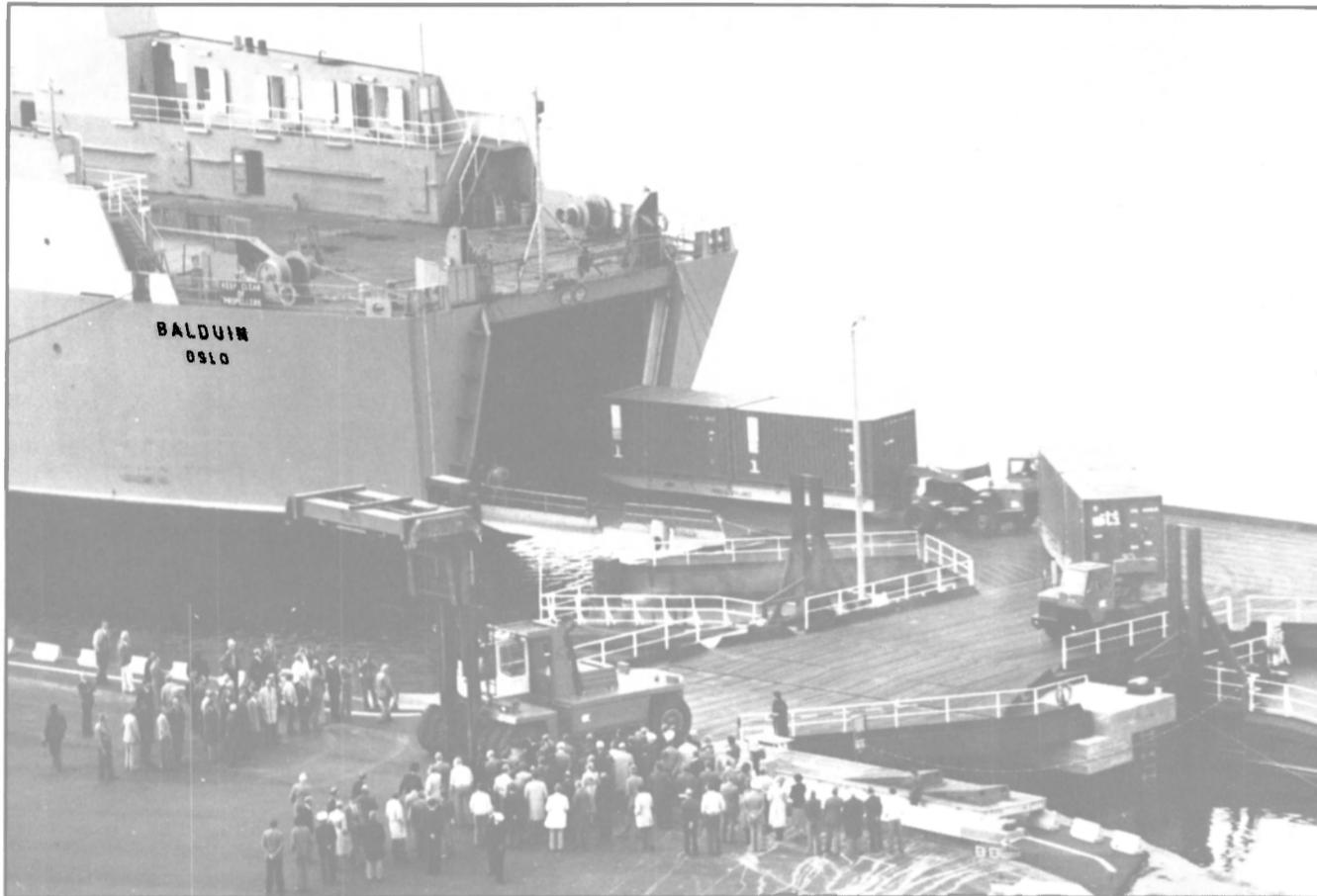
As more Ro-Ro ships enter service, demands for berthing facilities are increasing. In the Port of Oslo, the considerable depth of water would require extensive and costly engineering works if permanent new piers were to be constructed. The Port has therefore chosen to use a floating link span which can easily be moved from one location to another within the Port to cope with varying requirements due to changes in the traffic pattern.
