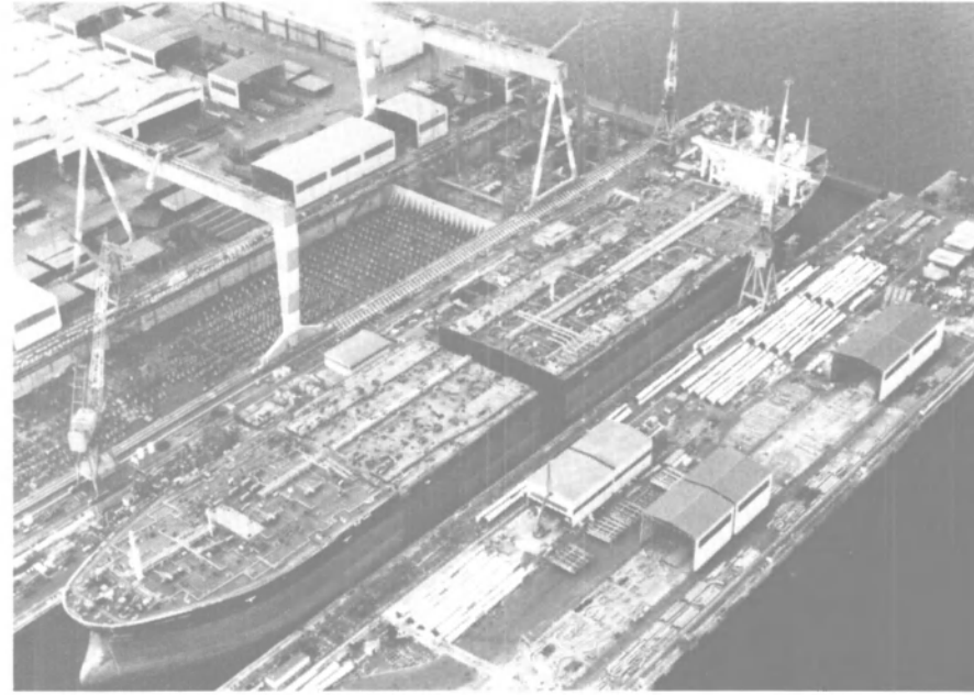
Insertion of a new 81-meter-long midbody added 140,000 dwt to the tanker Seawise Giant making her, at 560,000 dwt, world's largest tanker. Conversion was performed at Nippon Kokan's Tsu Shipyard in Japan for Universal Petroleum Carrier Inc.
