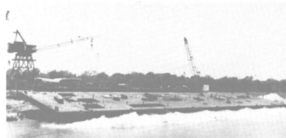
Side launching of 330-foot hull for a floating grain transfer facility took place recently at Bergeron Industries' yard in Braithwaite, La.
