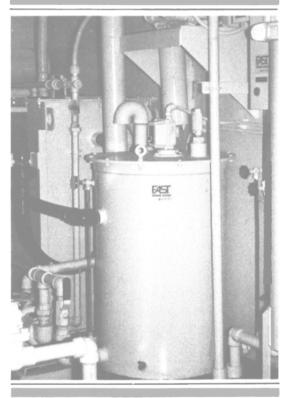
rugged in design, there are no adjustments. It operates with minimum maintenance, low operating costs and produces superior effluent quality. Available three ways: modular, completely assembled or built into vessel tankage. Accommodates 3 to 3000 persons. The FAST System is also convertible to Type III No Discharge operation if desired.
