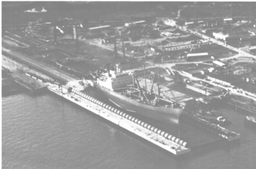
25,000 DWT vessel on platform awaiting transfer.
